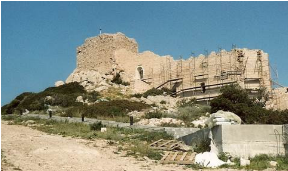
Kastellos under restaurering
